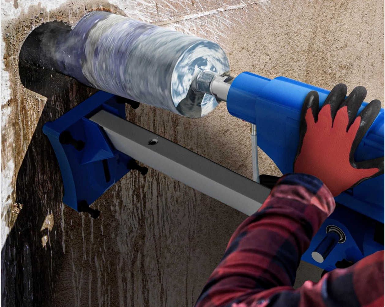
Figure 5.3: Dry drilling operation.
