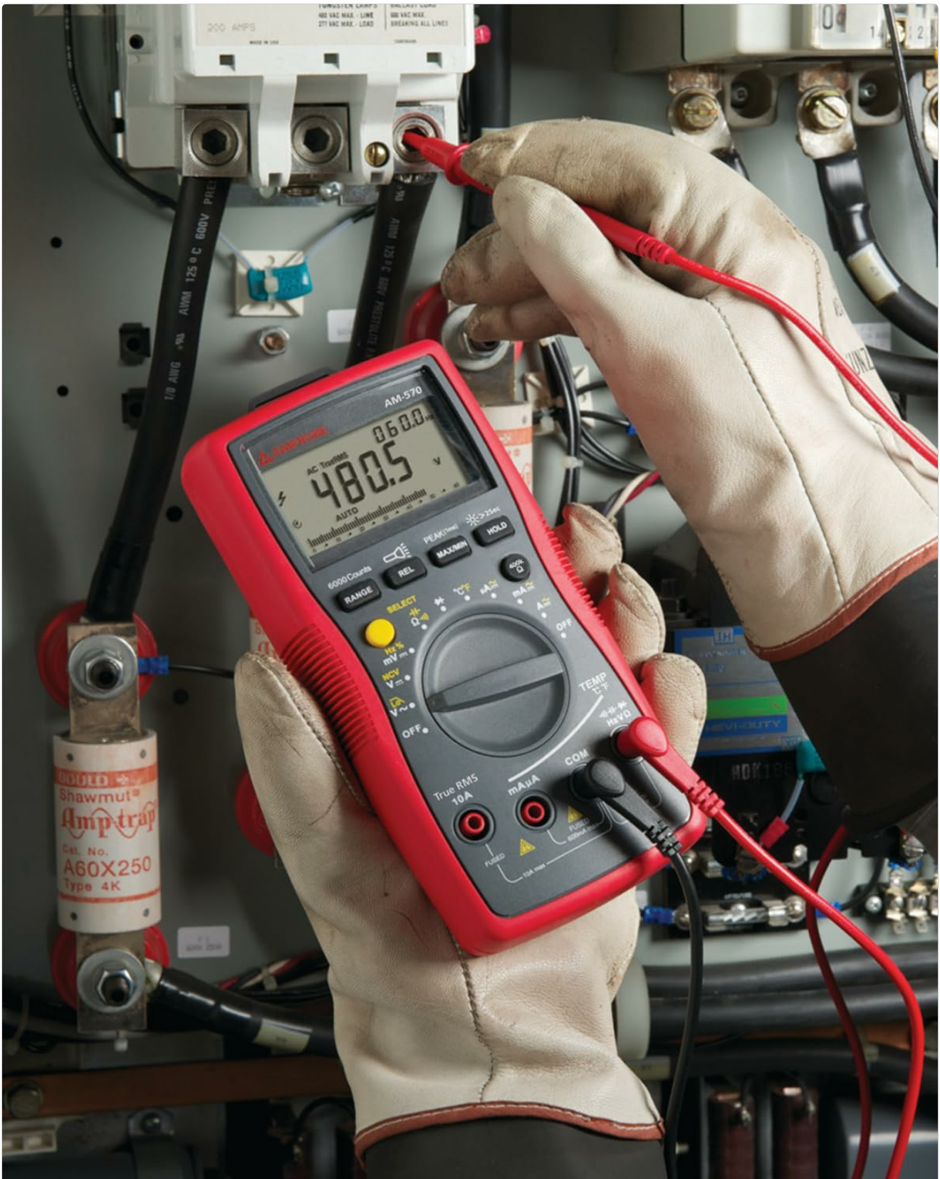
Image 6.1: An electrician utilizing the Amprobe AM-570 Digital Multimeter to perform voltage measurements within an industrial electrical panel, demonstrating practical application.
