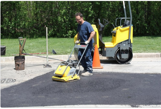
Figure 2: An operator guiding the WP1550AW compactor over a fresh asphalt patch, demonstrating typical usage in a construction setting.
