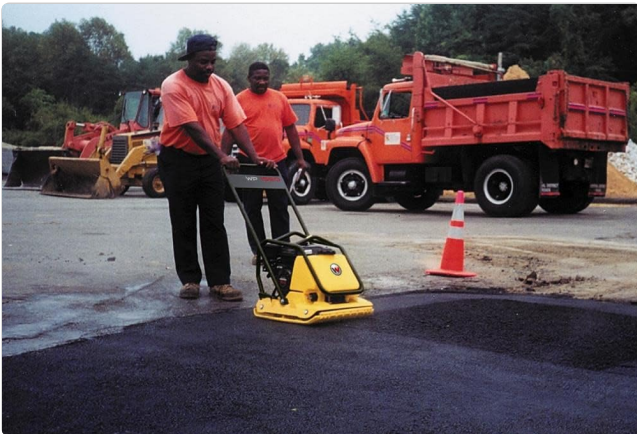
Figure 3: Two individuals working together to compact an asphalt surface with the WP1550AW, highlighting its maneuverability and ease of use.
