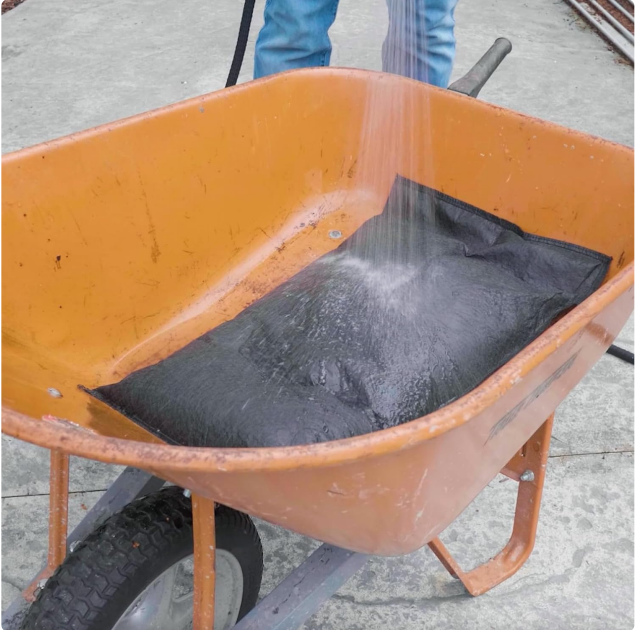
Image: A person pre-soaking a Quick Dam flood bag in a wheelbarrow using a garden hose. This demonstrates how to activate the bag before placing it in position.
