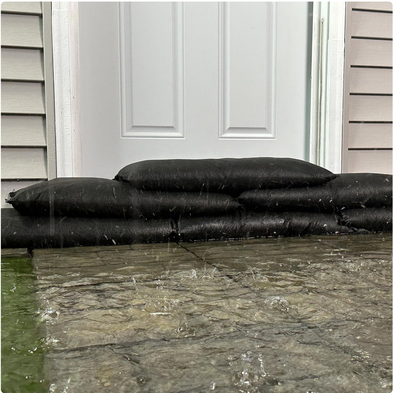
Image: Activated Quick Dam flood bags stacked in front of a house doorway, effectively blocking rainwater from entering.
