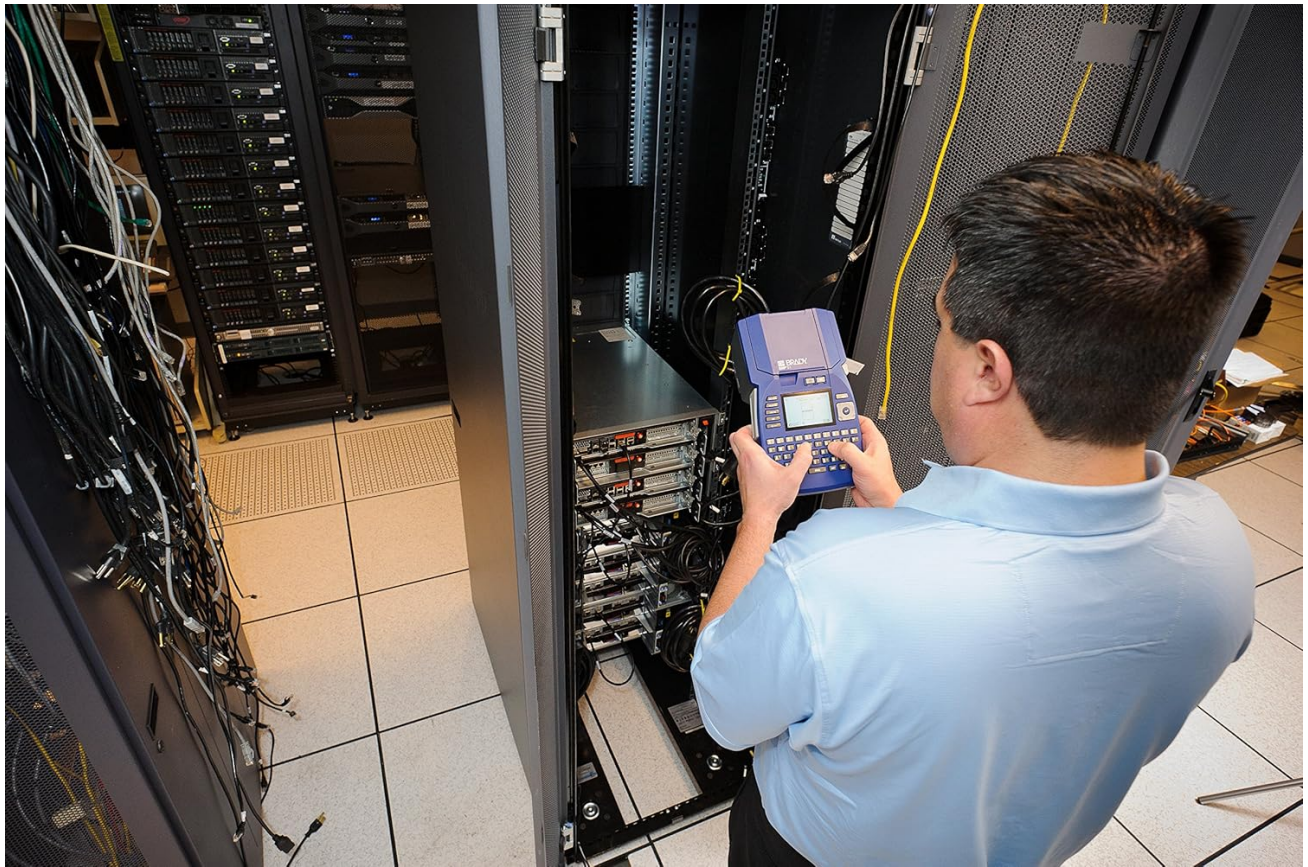
Figure 4.1: A technician operating the Brady BMP51 label maker to create labels for equipment within a server rack, demonstrating its portability and ease of use in field applications.
