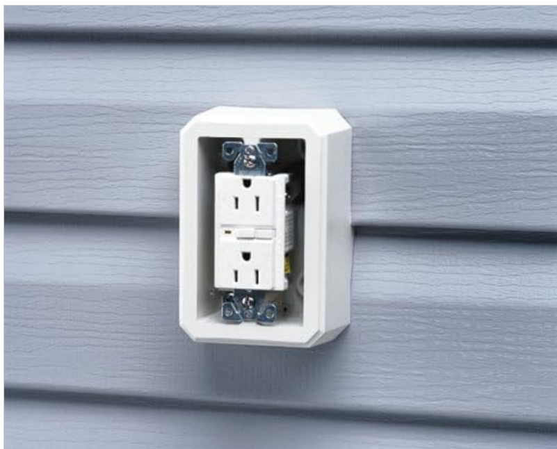
Figure 2: Electrical outlet fully installed within the FS8171 box.
