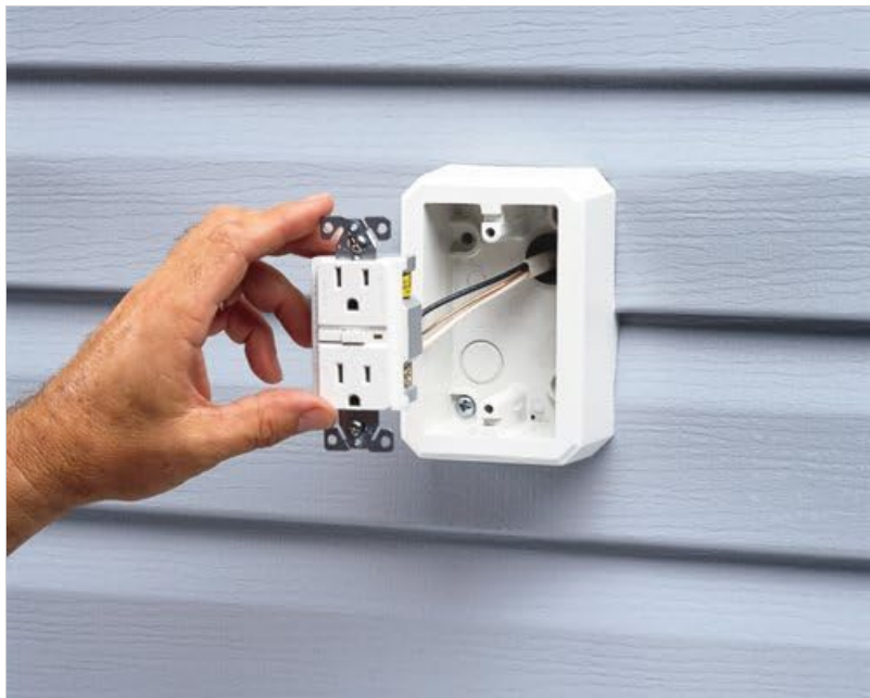
Figure 1: Inserting an electrical outlet into the mounted FS8171 box.
