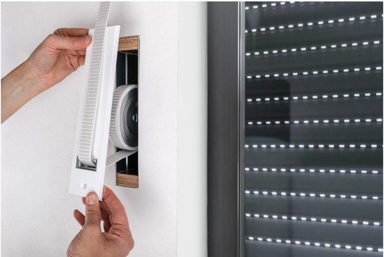
Figure 3: Illustrates the process of installing the winder into the wall box.
