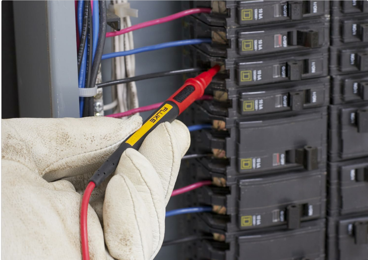
Figure 4: Using a Fluke TL175 Test Lead in a circuit breaker panel, demonstrating a CAT IV application with the shroud retracted.
