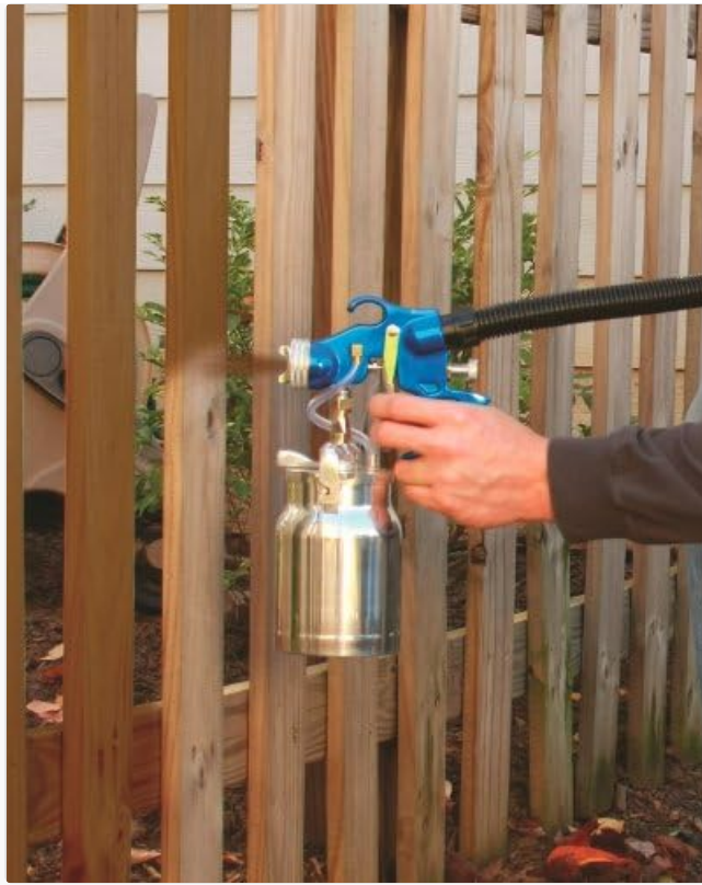
Figure 6: Efficiently coating a wooden fence with the HV5500 for even coverage.
