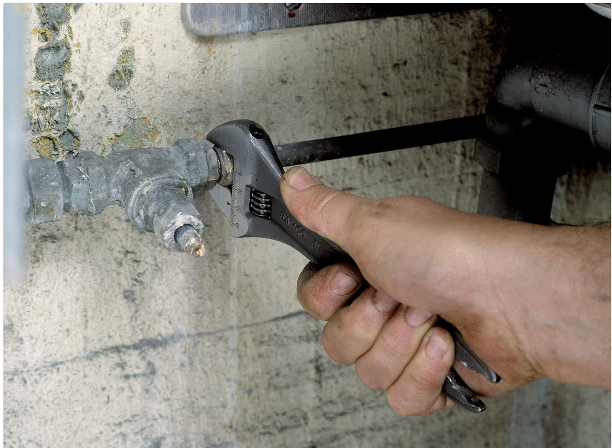
Figure 2: Adjustable Jaw in Use. This image shows a hand using the adjustable jaw of the wrench to turn a pipe fitting, demonstrating proper engagement.
