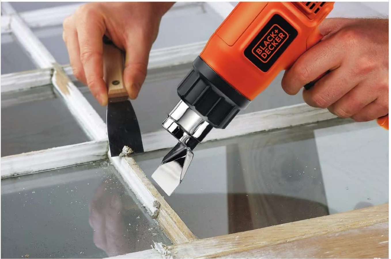
Figure 4: Using the heat gun to strip paint from a window frame.
