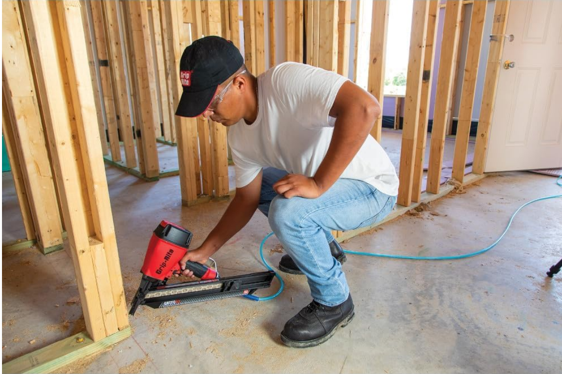
Figure 4.1: A user demonstrating the operation of the framing nailer on a wooden stud, highlighting proper handling and positioning.
