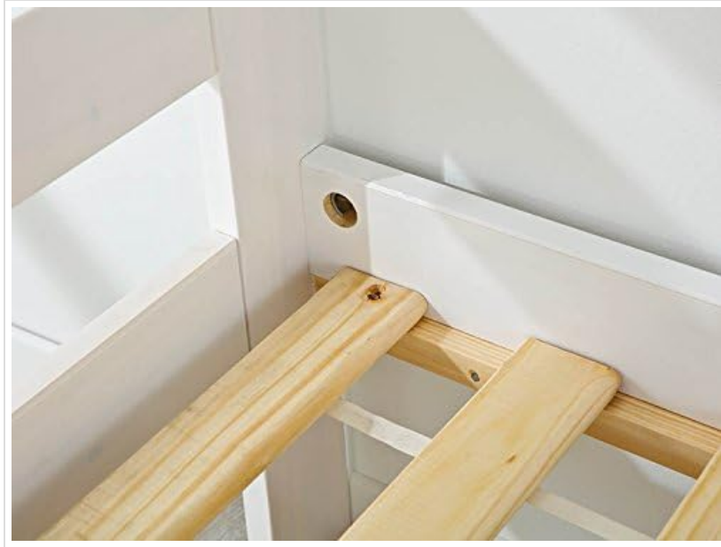
Image 3.2: Detail showing how bed slats are attached to the inner ledge of the side rail, providing support for the mattress.
