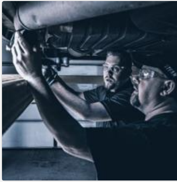
Image: Two individuals collaboratively working on an exhaust system, highlighting the potential need for assistance during installation.
