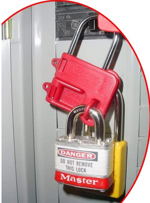
Image 4.2: Example of a lockout hasp securing an electrical installation, preventing accidental re-energization during maintenance.
