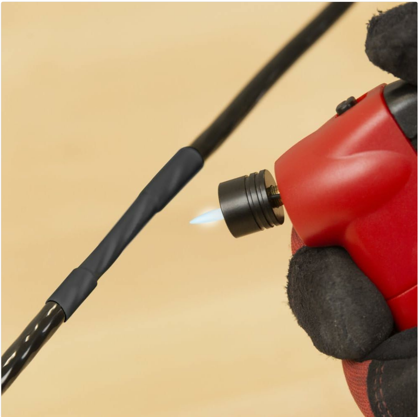
Figure 4: Applying heat to shrink the tubing securely around the wire.
