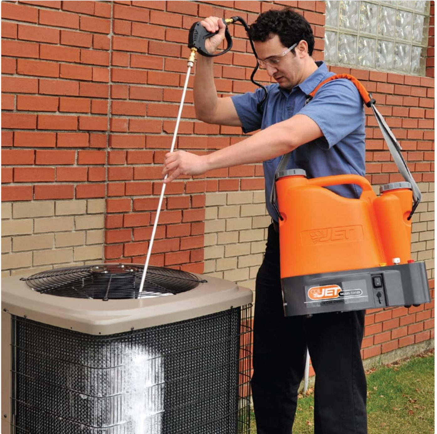
Image: An outdoor condenser unit is being cleaned by a technician using the SpeedClean CoilJet. The portable unit is worn with a shoulder strap for ease of movement, allowing access to all sides of the coil.
