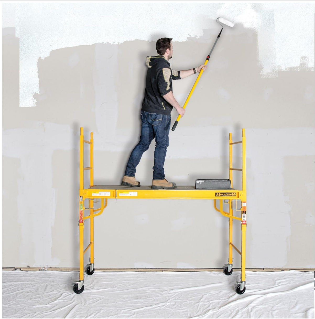
Figure 4.1: A user demonstrating painting from the stable MetalTech scaffolding platform.
