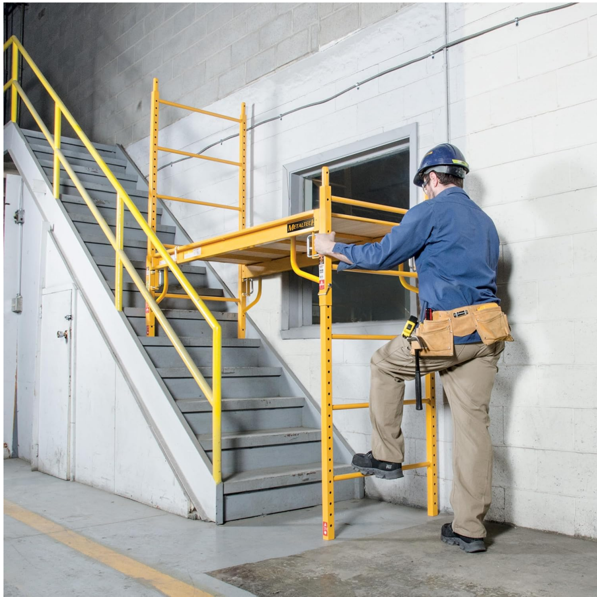
Figure 4.3: Scaffolding positioned on a staircase, demonstrating its adaptability for uneven surfaces.
