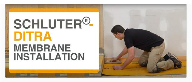
A person applying thin-set mortar to a subfloor using a notched trowel, preparing the surface for the DITRA membrane installation.
