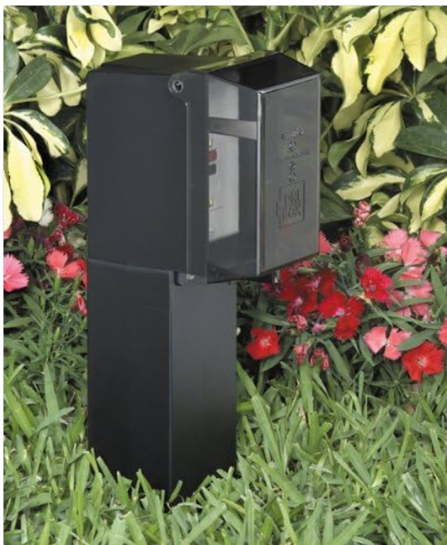
Figure 2: An ARLINGTON Gard-N-Post (similar model in black) installed within a garden, demonstrating how it blends with landscape elements. The outlet cover is open, revealing an installed electrical receptacle.
