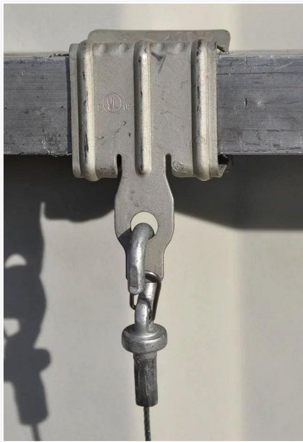
Figure 3.2: The Erico 4H24 clip attached to a flange, supporting a chain.
