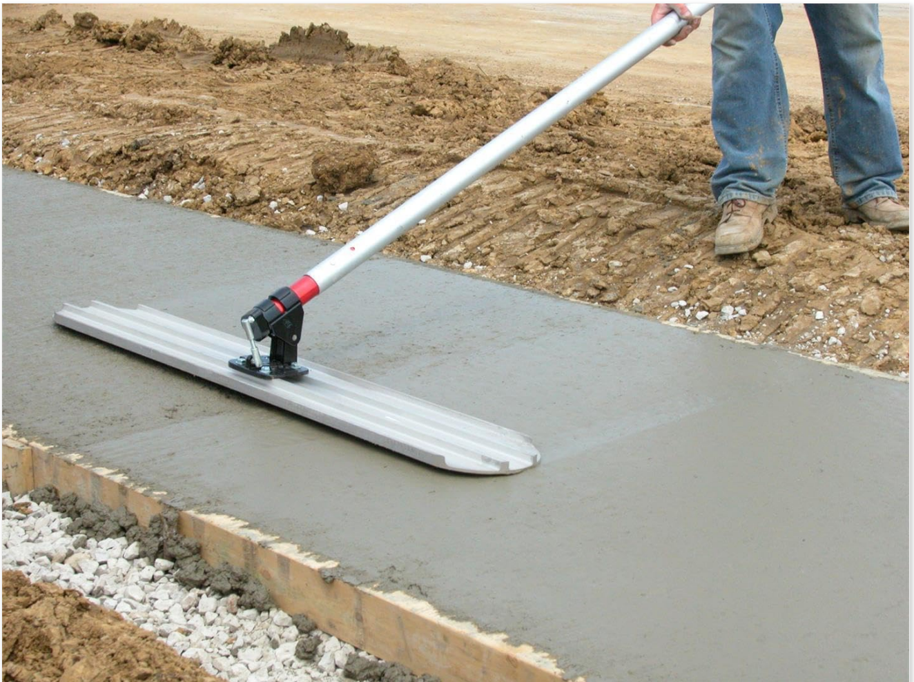
The bull float being used on a concrete slab, demonstrating its function in leveling and smoothing the surface.
