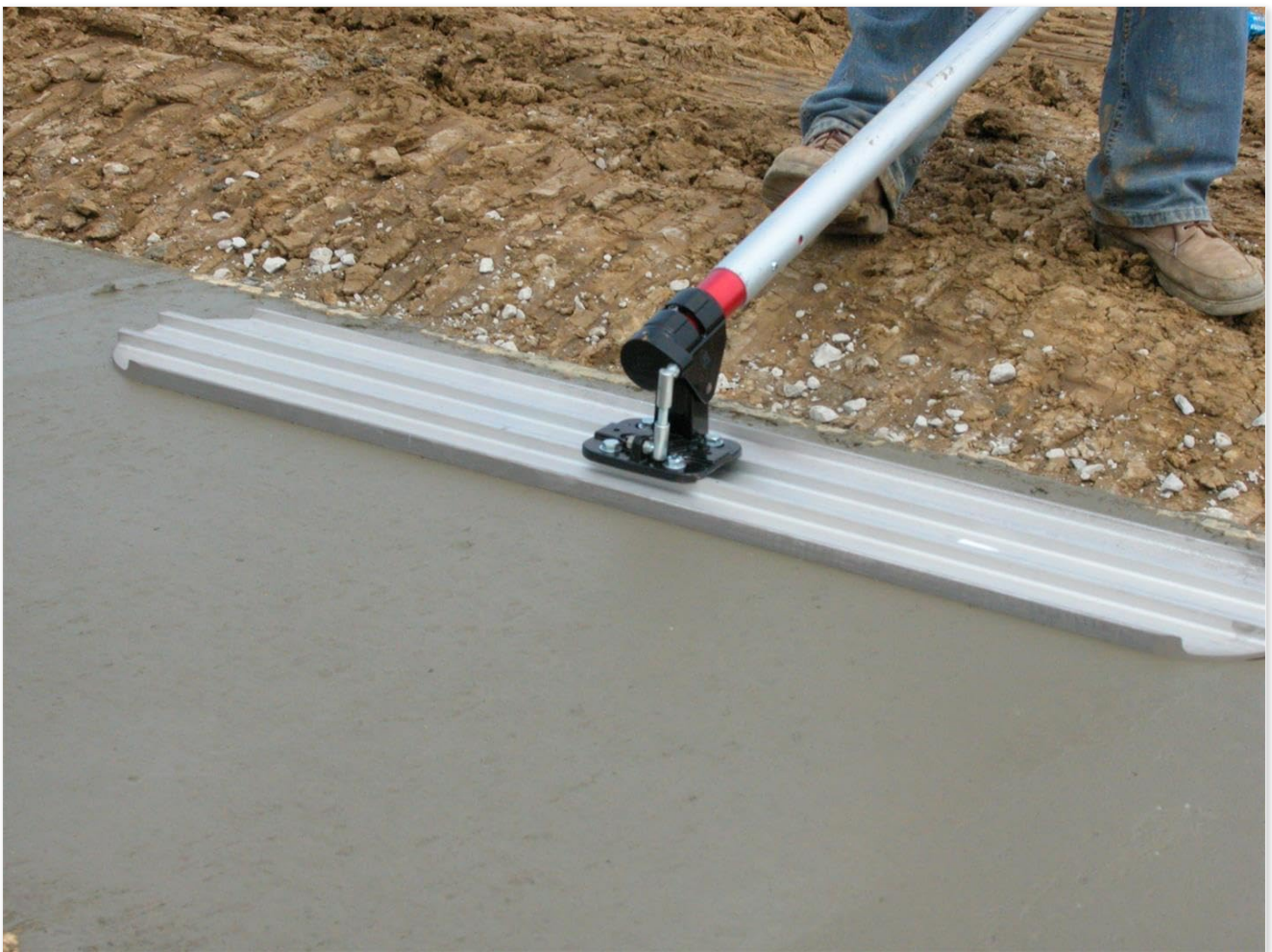
Top-down view of the bull float and its bracket, showing the connection point for the handle.
