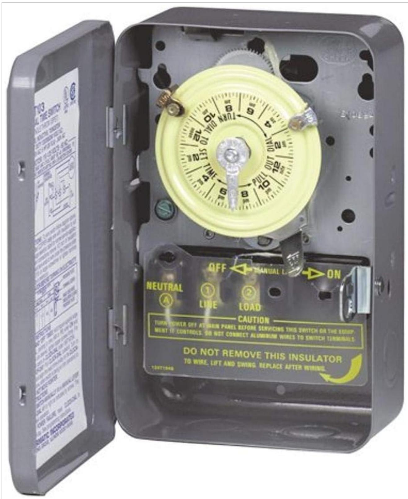
Image: The Intermatic T102 mechanical time switch with its metal enclosure door open, revealing the yellow 24-hour dial, the manual override lever, and the wiring terminals (Neutral, Line, Load). A warning label regarding aluminum wires is visible at the bottom.
