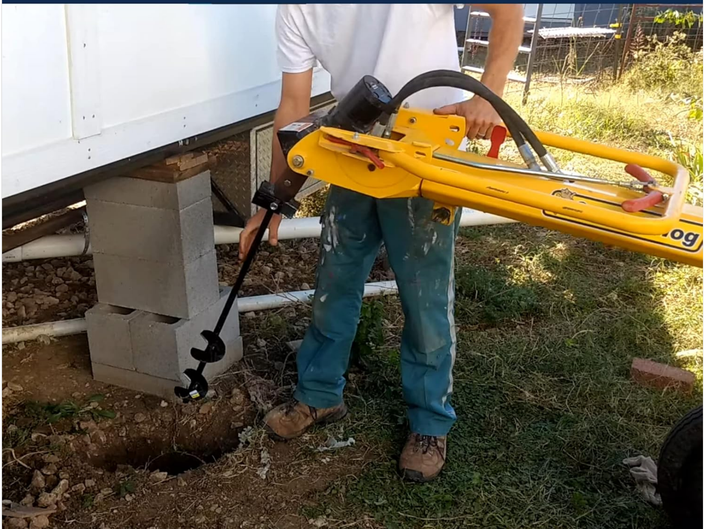
Figure 6: Example of earth anchor installation using a driving tool.
