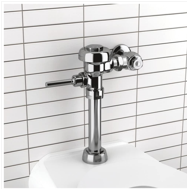
Figure 4: The Sloan Regal 111 Flushometer shown installed on a water closet, illustrating its integration with the fixture.
