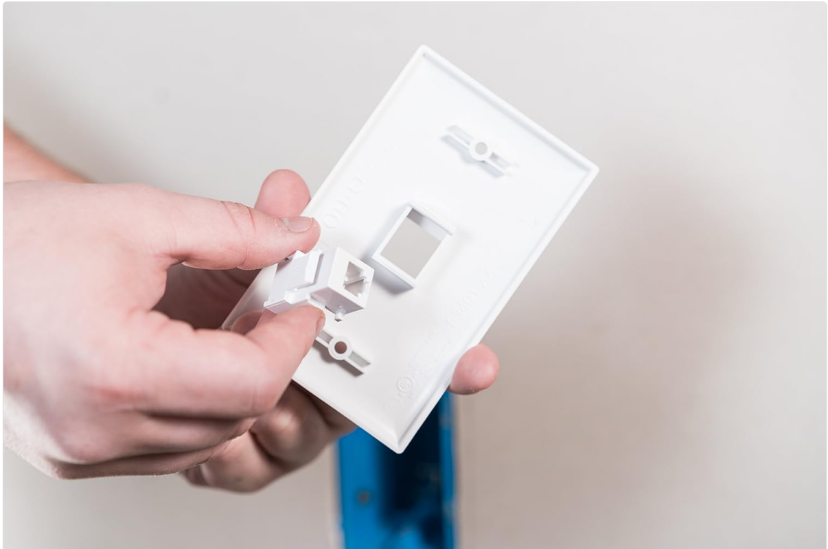
Figure 4: Inserting the keystone jack into a compatible wall plate opening.
