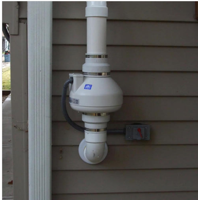
Figure 3.3: Example installation of the RadonAway RP145c Radon Fan on an exterior wall. The fan is integrated into a PVC pipe system, demonstrating a typical setup for radon mitigation, with the fan positioned vertically between two pipe sections.
