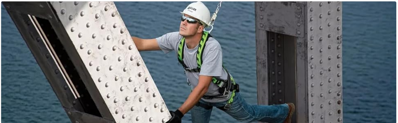
Image: A worker demonstrating the proper wearing of a fall protection harness in an industrial setting.
