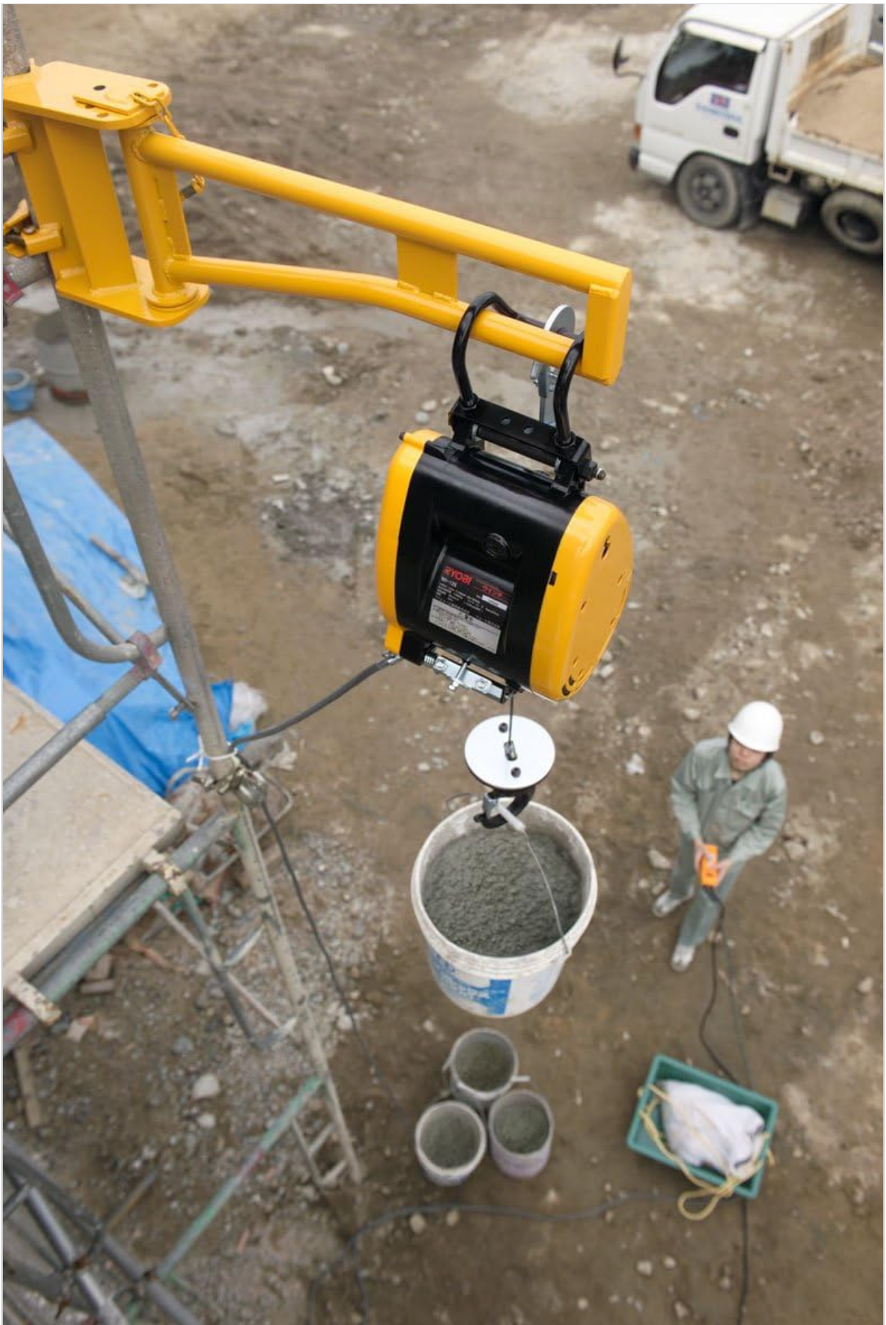
Image: A close-up view of the Kyocera WI-125 Electric Winch lifting a bucket filled with construction material. The winch is mounted on a yellow arm.
