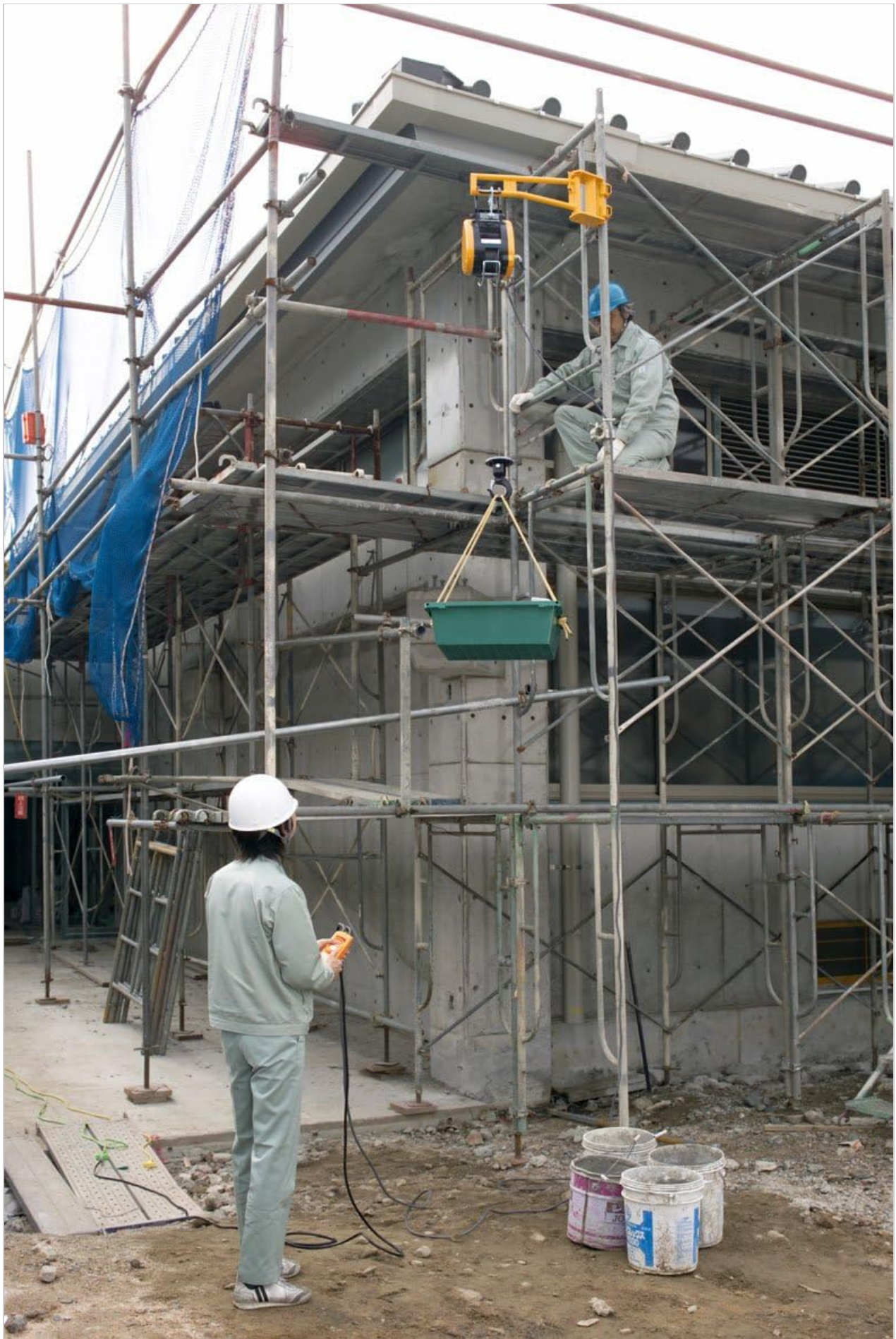
Image: Kyocera WI-125 Electric Winch being used to lift materials on a construction site. A worker operates the remote control while another worker is positioned higher up.
