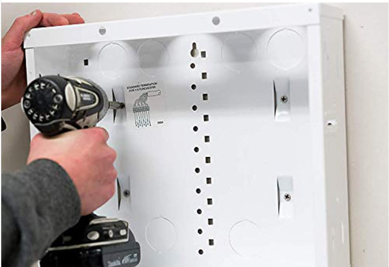
Figure 3.1: Securing the enclosure to wall studs during installation. The enclosure can be recessed or surface mounted.
