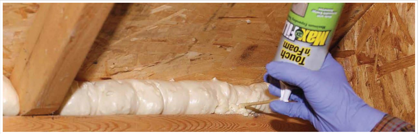
Image: A person wearing gloves applying DAP Touch 'n Foam Max Fill into a gap between wooden beams, demonstrating typical application.
