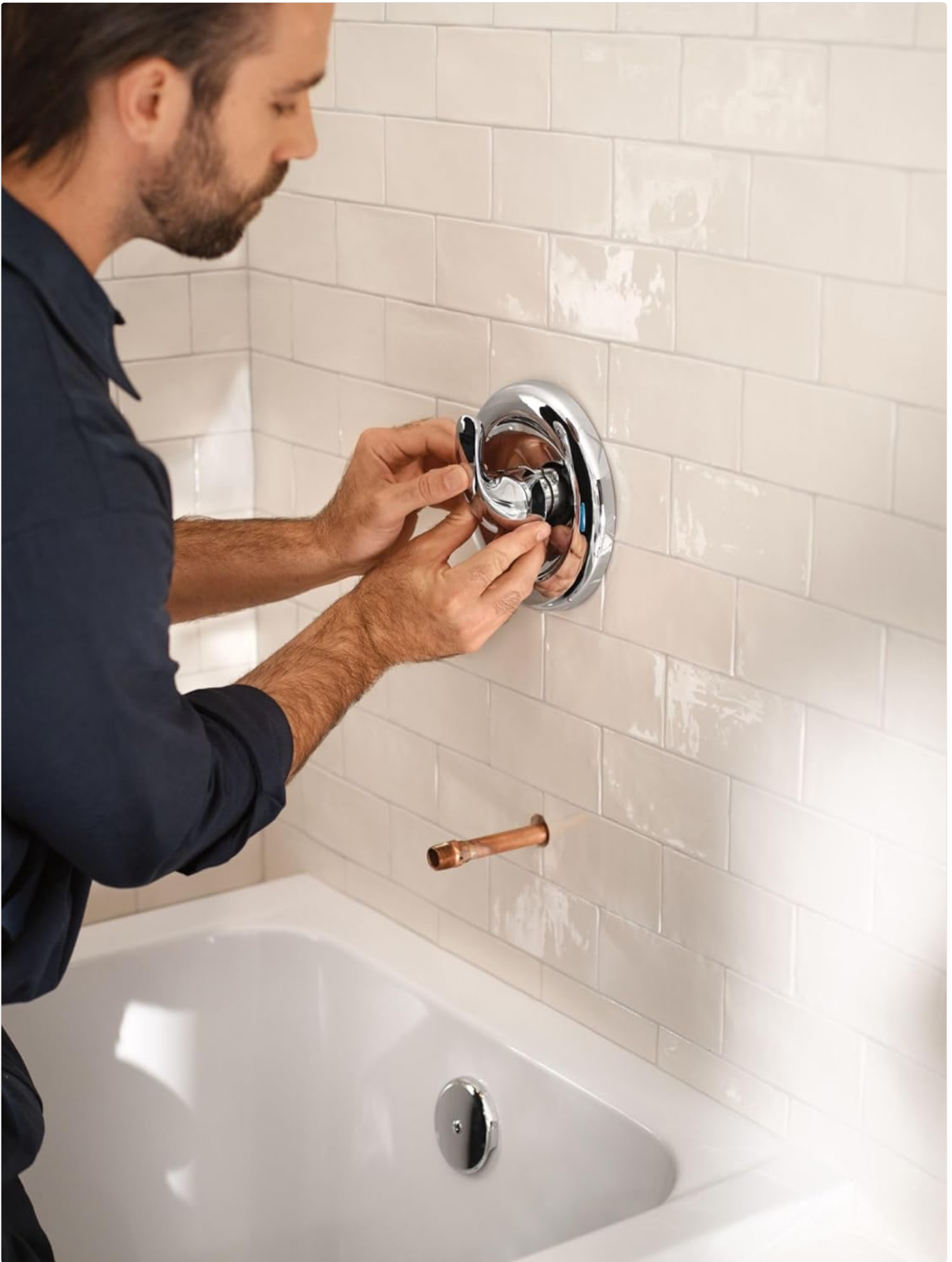
Image: A person installing the decorative trim kit over a Moen PosiTemp valve, demonstrating the ease of finishing the installation.
