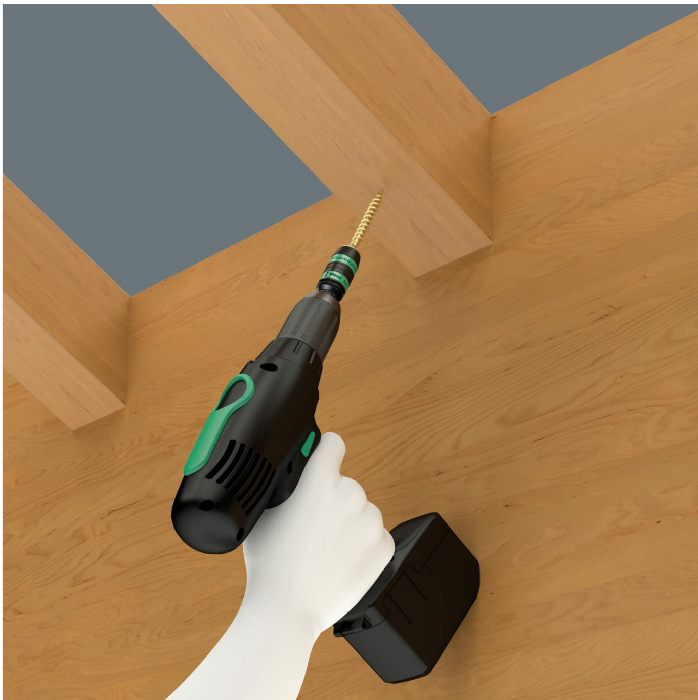
Figure 6: Screw held securely by the ring magnet.
