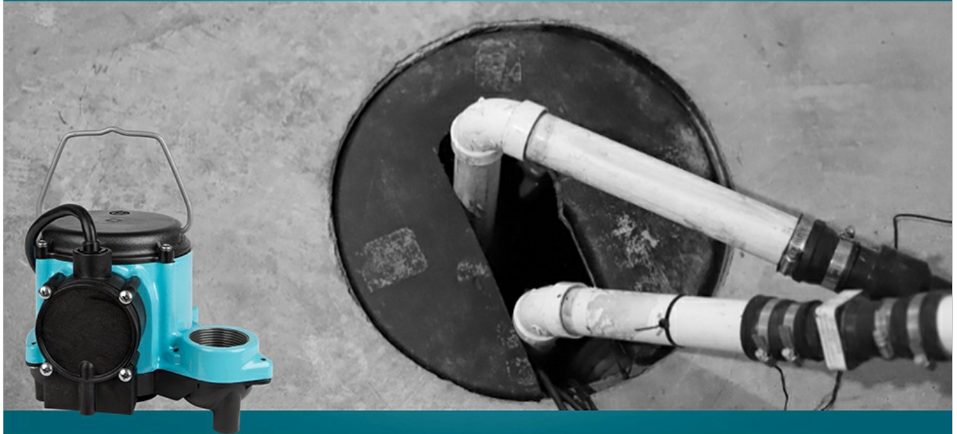
Image: Little Giant 6-CIA Sump Pump installed in a basement sump pit, illustrating typical application. The pump is submerged in water within the pit, with discharge piping extending upwards.
