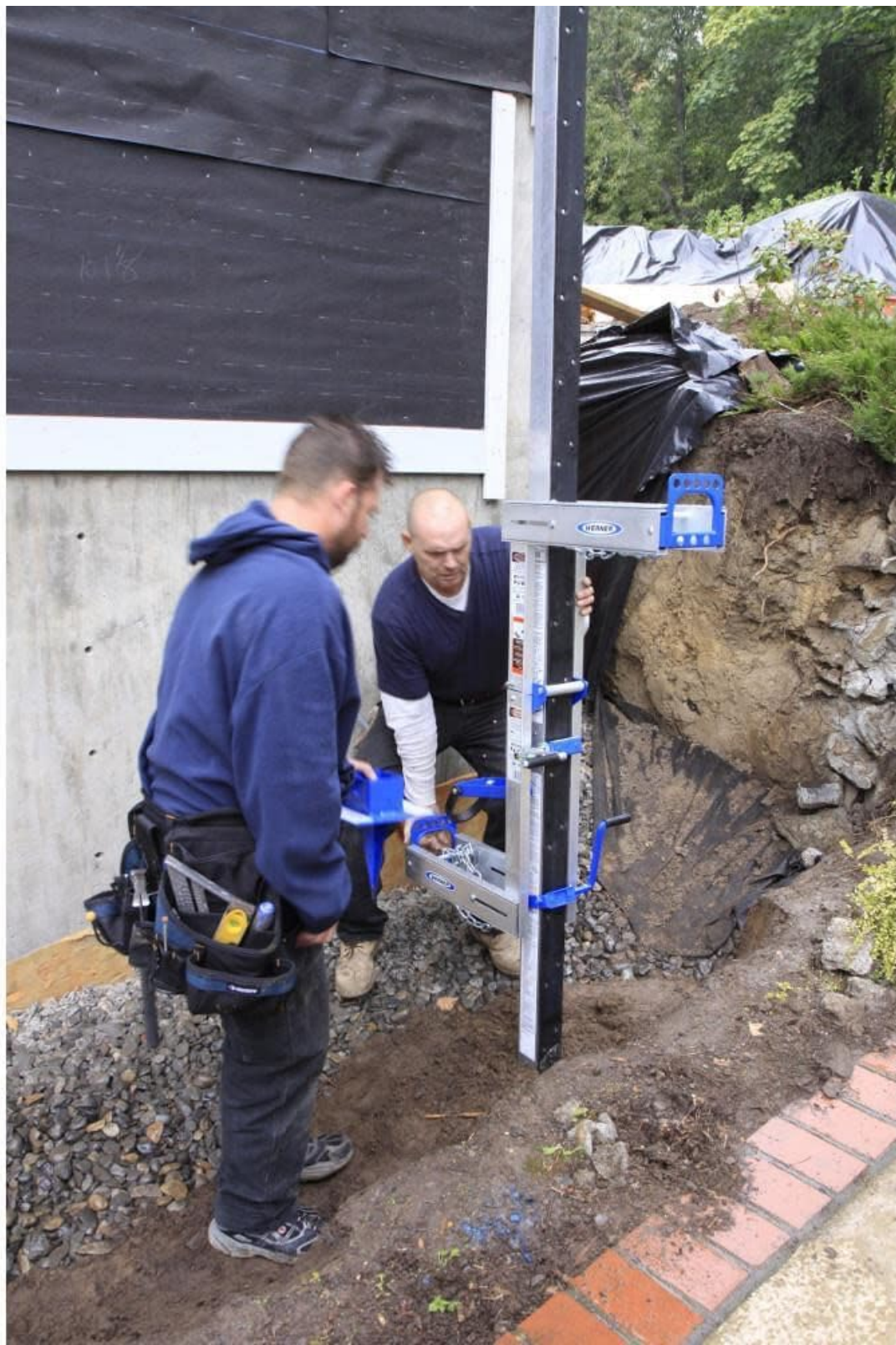
Image: Two workers installing a Werner pump jack unit onto a vertical support pole, ensuring proper alignment and secure attachment.
