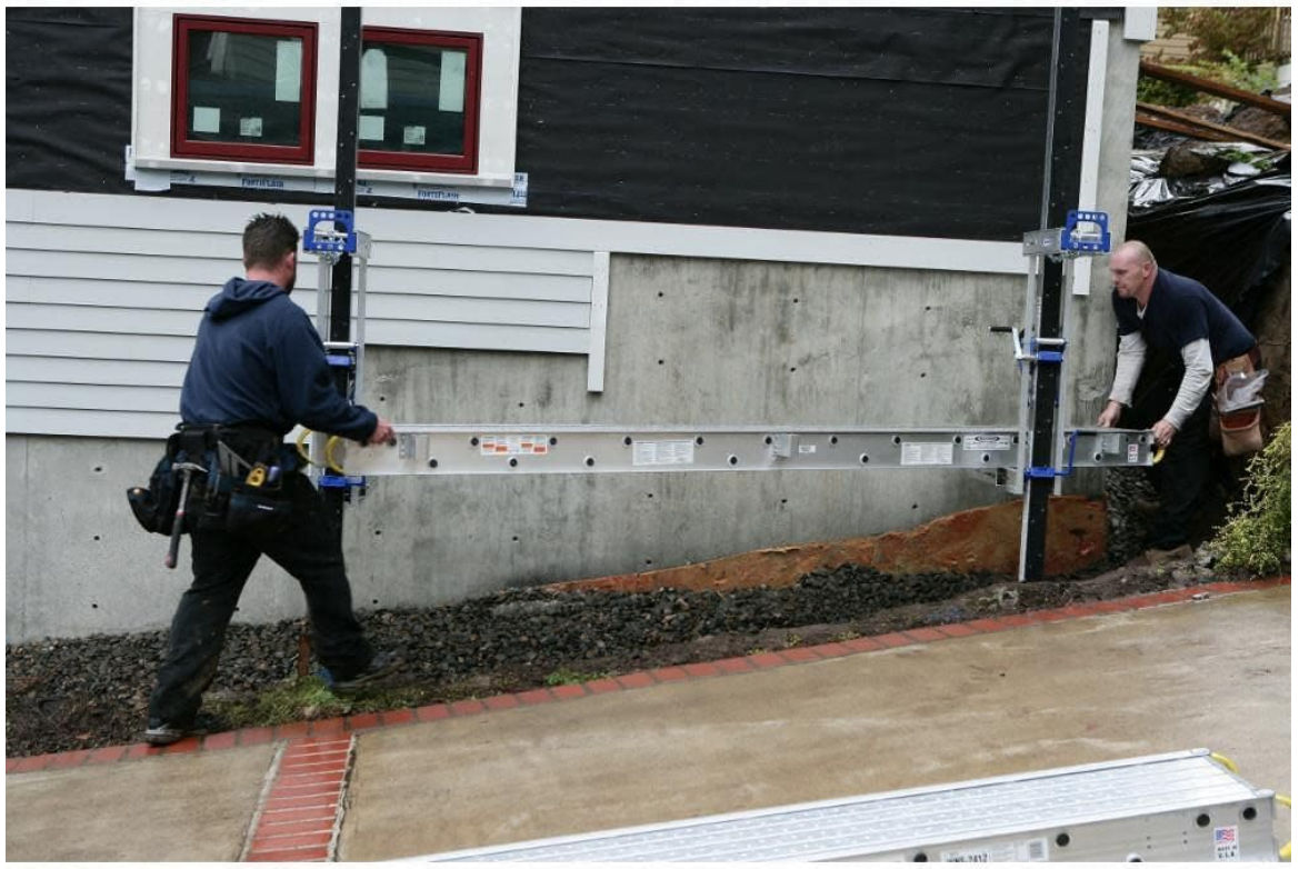
Image: Two workers carefully positioning a long staging plank onto two installed pump jack units, ensuring even distribution and secure placement.
