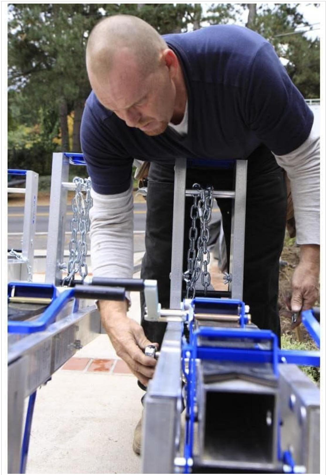
Image: A worker securing a chain on the pump jack unit, demonstrating a critical step in ensuring the stability and safety of the assembly.
