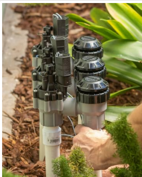
Image 4: Close-up view of the solenoid being screwed into the valve body, illustrating the
