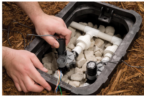
Image 2: A person's hands installing a new solenoid into an irrigation valve within a valve box. This demonstrates the typical installation environment.
