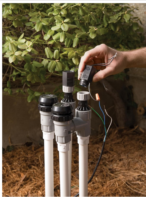
Image 3: A hand holding the solenoid, showing the attached wires ready for connection. This highlights the electrical connection step.
