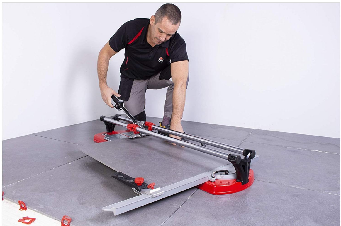
Figure 6: A user applying downward pressure on the handle to activate the breaker mechanism, cleanly separating the tile along the scored line.
