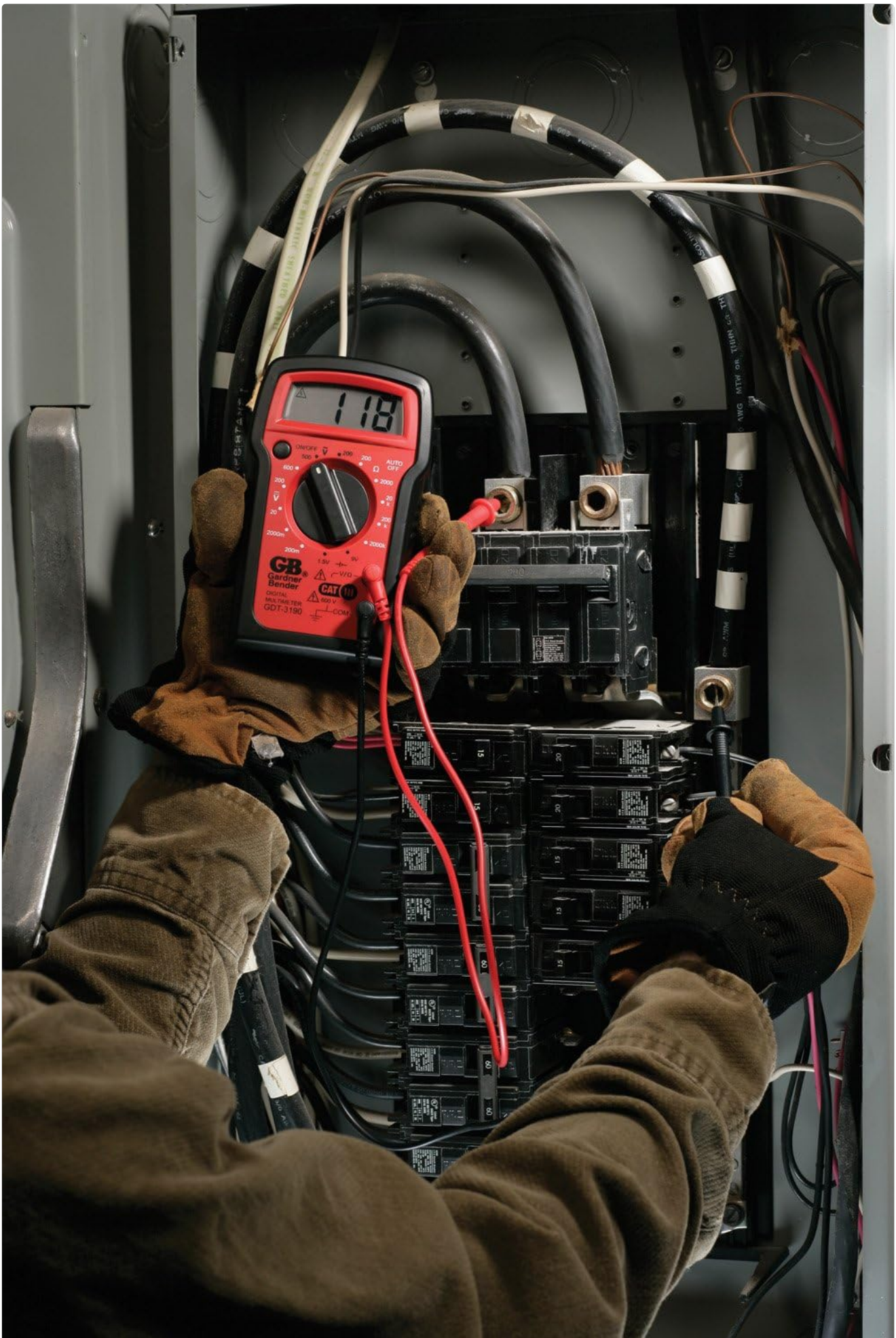
Figure 3.3: Measuring voltage within a circuit breaker panel using the multimeter.
