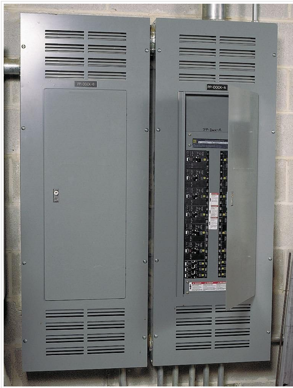
Image: Two Schneider Electric panelboards, one with an open cover showing circuit breakers.
