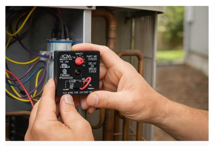
Hands installing the ICM Controls ICM203 Delay on Break Timer into an HVAC unit, showing wiring connections.
