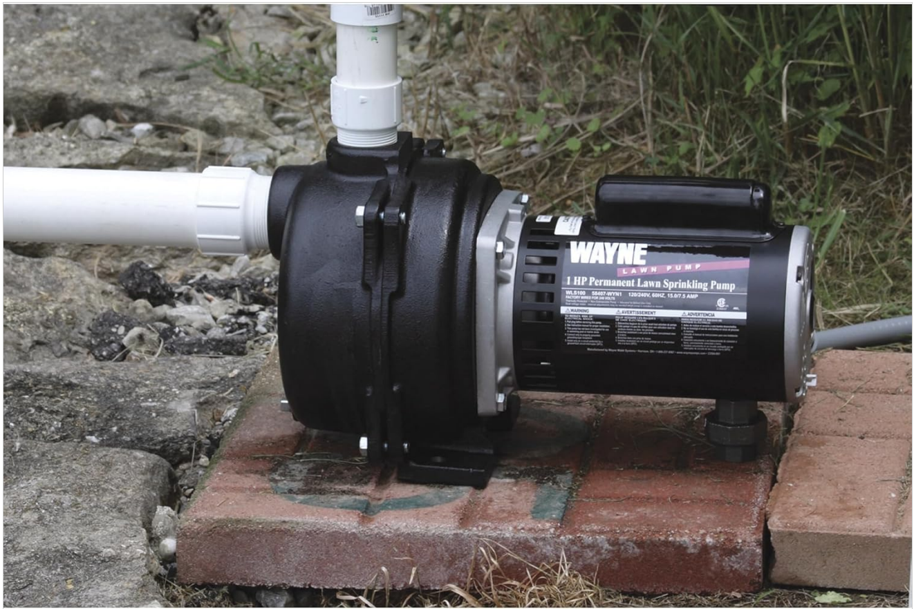
Image 4.1: Example installation of the WAYNE WLS200 pump with PVC piping connections.
