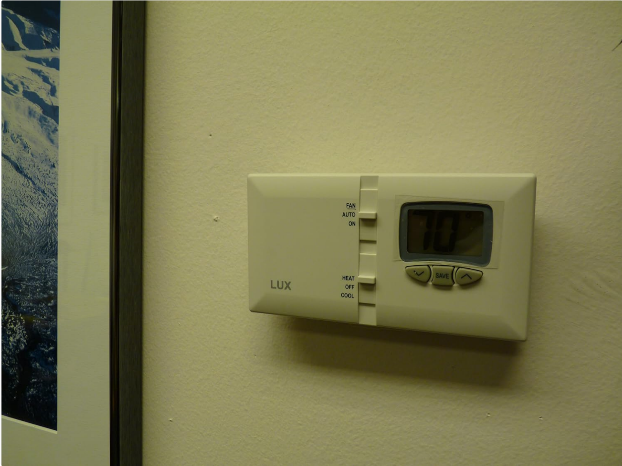
The thermostat installed on a wall.
