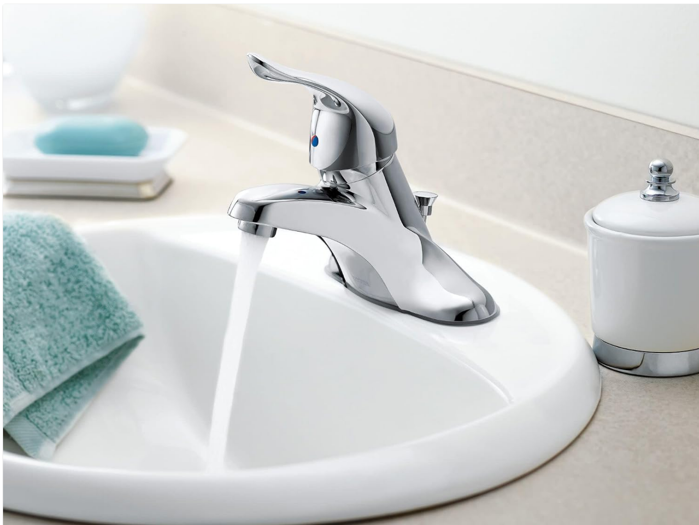
Figure 3: Faucet installed and in operation.
