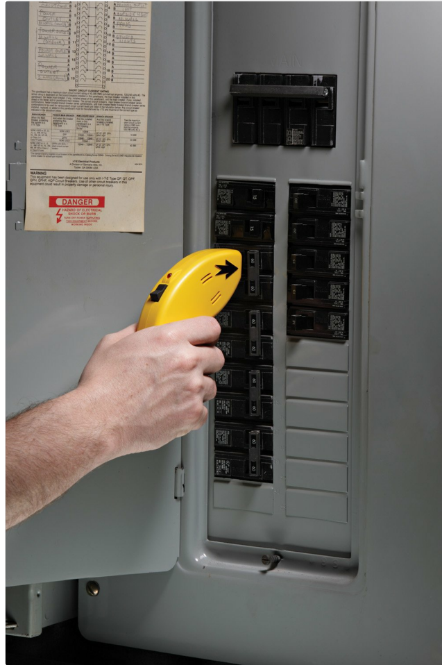
Image: The receiver unit being used to scan circuit breakers within an electrical panel.
