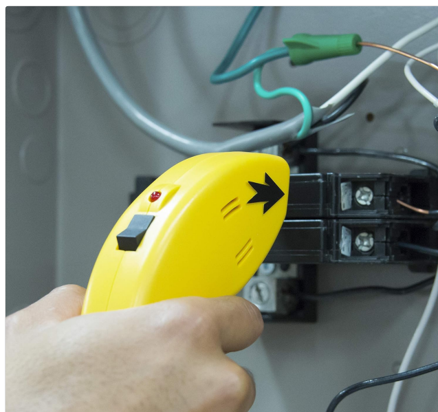
Image: A close-up view of the receiver indicating the correct circuit breaker with its LED light.
