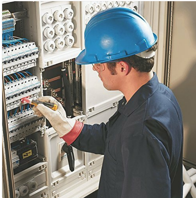
Image: An electrician using the Fluke 1AC II VoltAlert to safely test for live circuits within an electrical panel.
