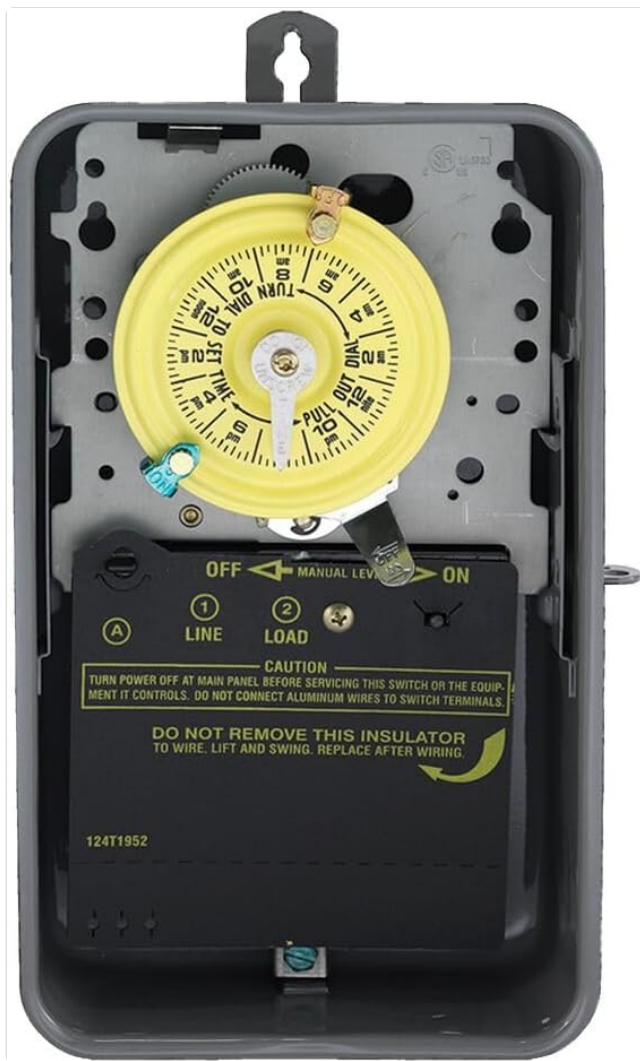
Figure 1: Internal view of the Intermatic T101R timer switch, displaying the yellow 24-hour dial and the manual override lever.
