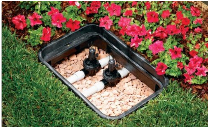
Figure 2: Example of a Toro sprinkler valve installed within an underground valve box. This illustrates how the valve is typically housed and connected to the irrigation system.
