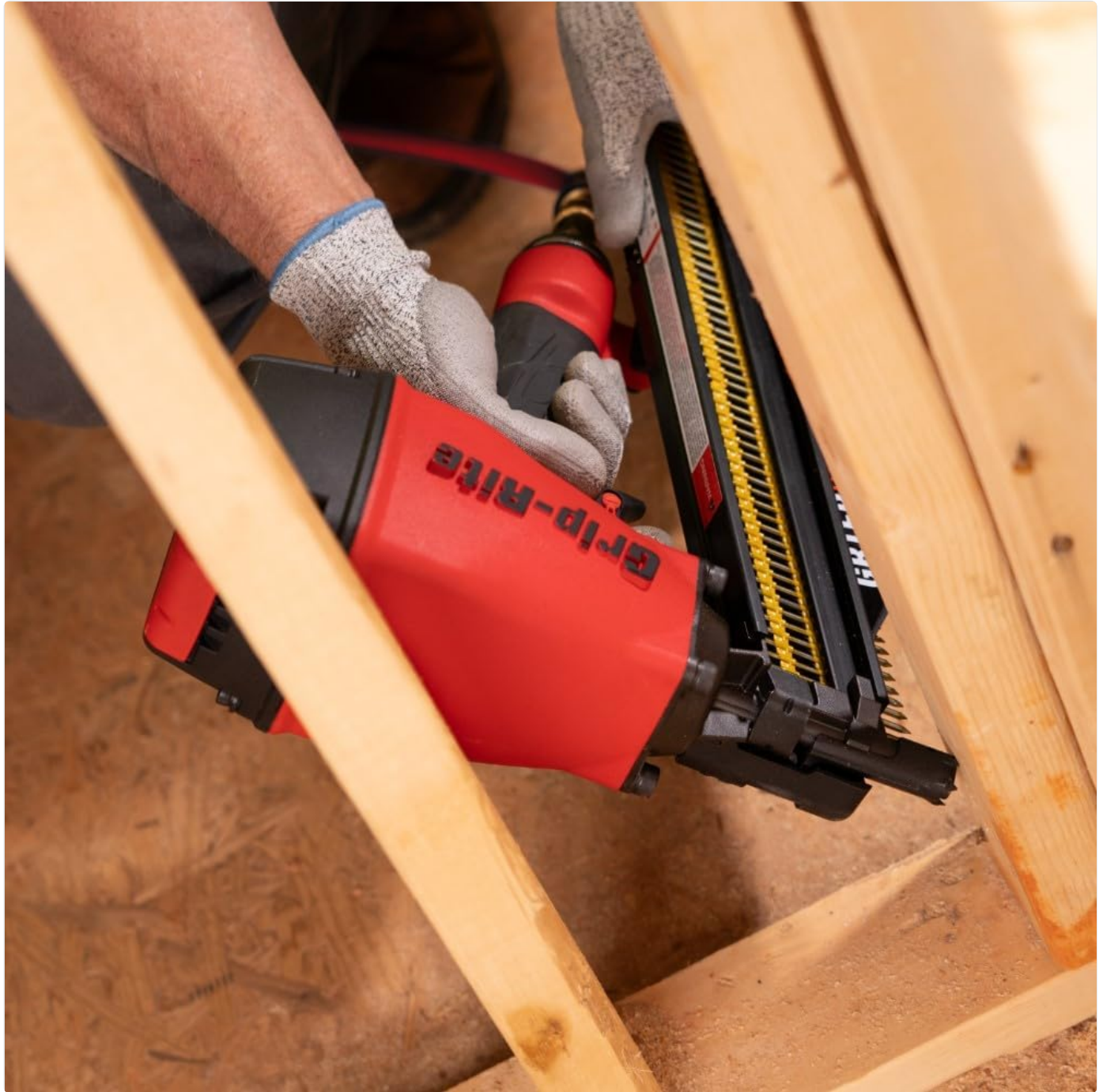
Image: A worker demonstrating the use of a framing nailer, likely loaded with Grip-Rite nails, to secure wooden framing in a confined area, highlighting the tool's maneuverability.
