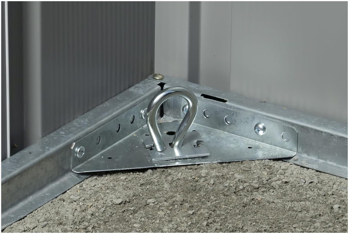
Image: A close-up of a shed corner showing the securely installed earth anchor and corner gusset on a concrete base.
