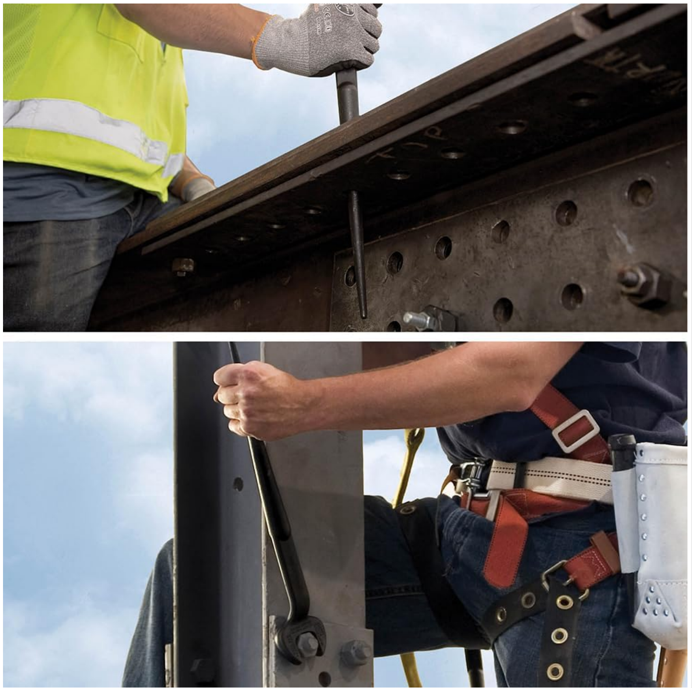
Figure 3: Demonstrating the use of the tapered handle for aligning bolt holes.
